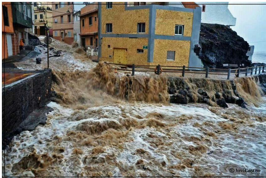
Flash floods in Güimar's municipality, December 2013 5
